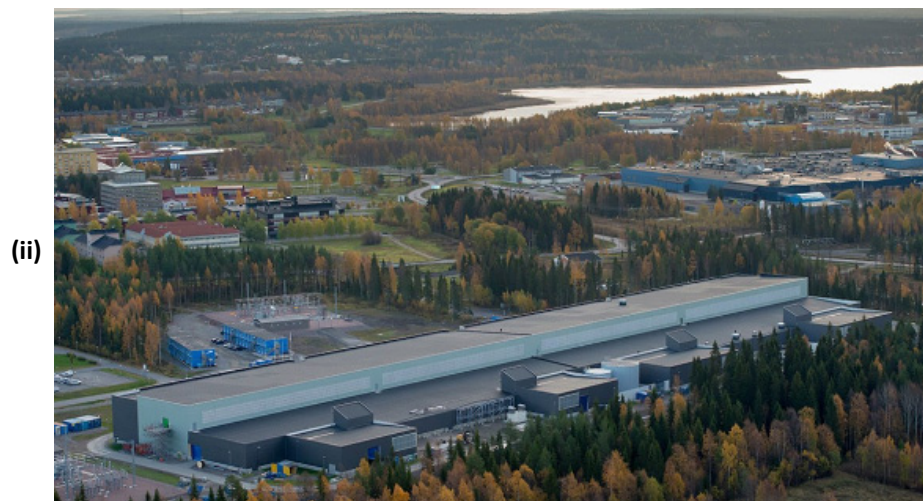
Facebooks serverhall (datacenter) i Luleå
